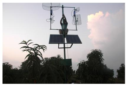
Figure CSD 7: Last touches to solar relay, Kumaon Network
