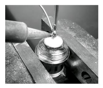
Figure AC 26: Solder the wire to the gold cup on the N connector. Insert a washer and gently screw the nut onto the connector. Trim the wire at 3.05 cm measured from the bottom part of the nut.
