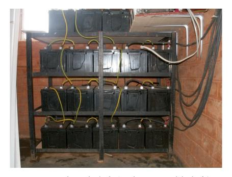
Figure OGP 9: A battery bank of 3600 Ah, currents reach levels of 45 A during charging
