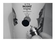
Figure AC 24: Carefully drill a pilot hole, then use a larger bit to finish the job.
