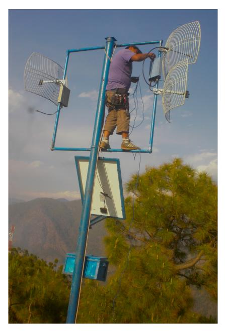
Figure CSD 8: Backhaul Relay, Garhwal Network
