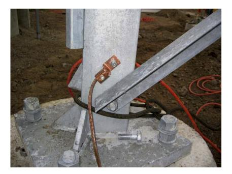
Figure HW 3: A tower with a heavy copper grounding wire.
