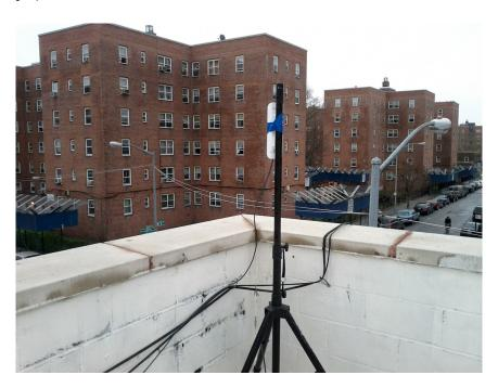
Figure CsOTI 4: First RHI WiFi node (Ubiquiti Nanostation) installed on the rooftop of the building that houses the RHI offices.
