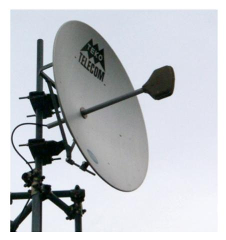
Figure ATL 14: A solid dish antenna.
